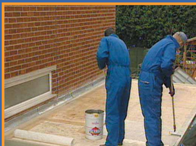
APPLYING THE NEW COMPOSITE
