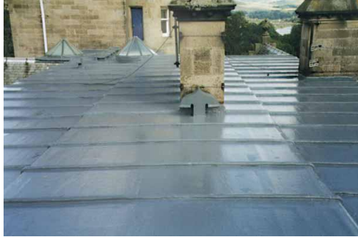
Elastex System applied to existing roof
