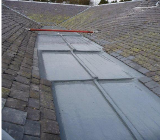
Elastex System applied to existing lead gutter
