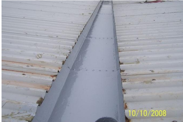
Elastex System applied to existing metal gutter
