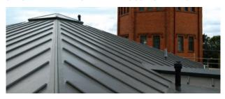
The aesthetics of this development were given the upmost importance after local planning constraints did not permit the use of traditional slate. After considering more expensive and vandal prone alternatives such as lead sheets, the client specified the BBA approved Polyroof 185 System with lead roll finish, which carries a 20 year insurance backed guarantee.
