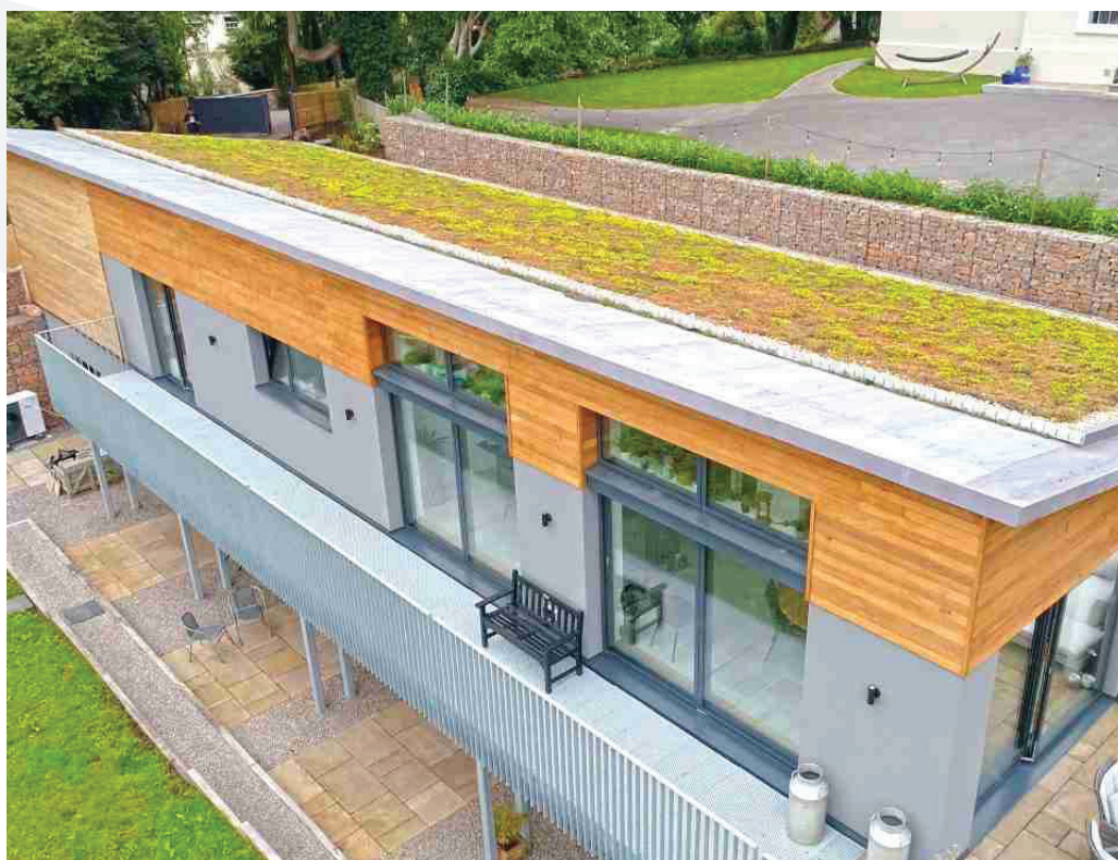
This new build 223m 2 roof, with a distinctive 10-degree mono-pitch rectangular shape, integrates a comprehensive green roof system, extended overhangs and onboard gutters. The design allows for the future installation of a photovoltaic array.
